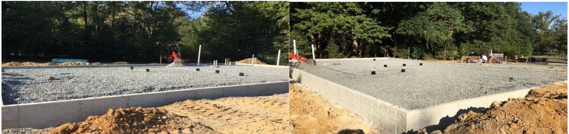
The Week of September 22 - Floor Drains, Bathroom Piping, Water/Sewer Line Connections
