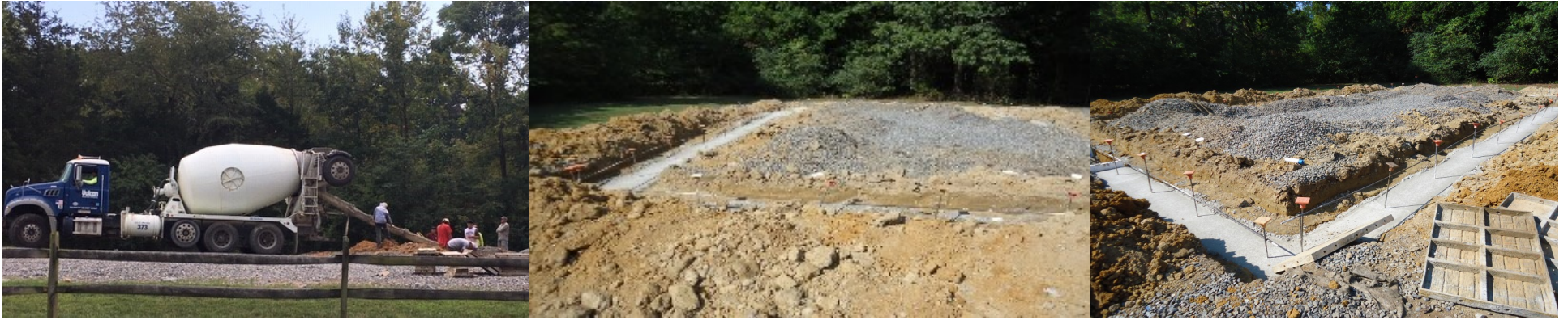
The Week of September 15th - Plumbing and Electrical Ground Works
